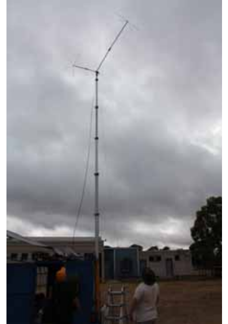
Up it goes, the compressed air mast ↑
