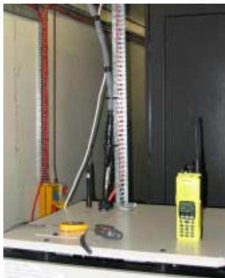
**Rail loop cabinet with MMR portable radio during rail loop underground testing. This portable is an MFB portable which is “intrinsically safe”.**
