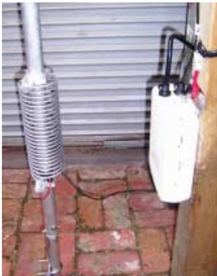
Some thicker dual walled 1.3 meter lengths of Aluminium tubing was used, placed at the rear yard via an Icom AH4 auto tuner, fed with 9913 coax (got to watch those dB losses at 160m!), with one radial along the back fence. The first mast length was 9 meters high, which did not tune below 80 meters.
